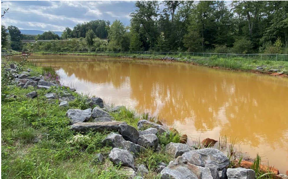
Figure 4-1: E41201637596786 "Askam Wetlands Maelstrom Oxidizer AMD Treatment System on Nanticoke Creek (outlet sampling)" looking at settling pond
