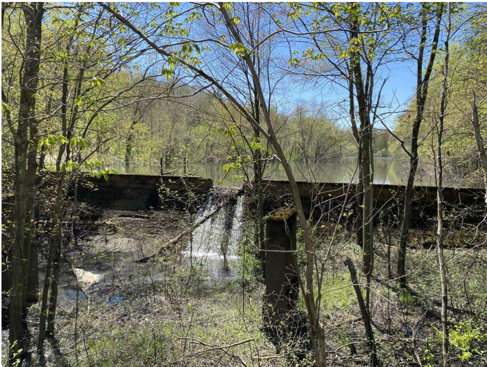
Figure 4-32: E41186777597290 "Leuders Creek Dam" looking at flow over the dam
