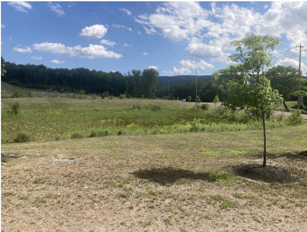
Figure 4-14: E41196737598797 "Espy Run Wet Stormwater Basins Vegetated" looking south at 2 wetlands separated by a berm (0.61 acre in the foreground and 0.75 acre in the background)
