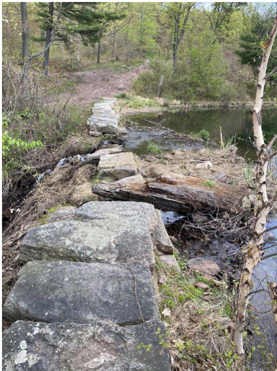
Figure 4-25: E41174187598896 "Hanover Reservoir" looking at dam
