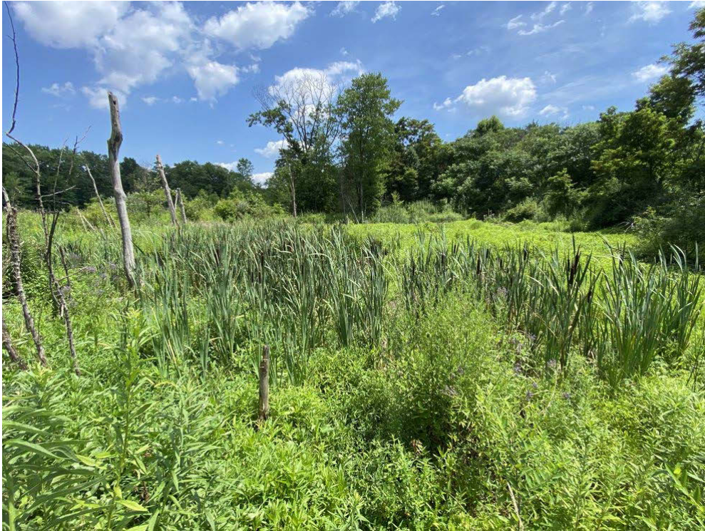
Figure 3-10: E41211367594534 "Below Hanover Crossing Road Culvert (M)" looking southeast
