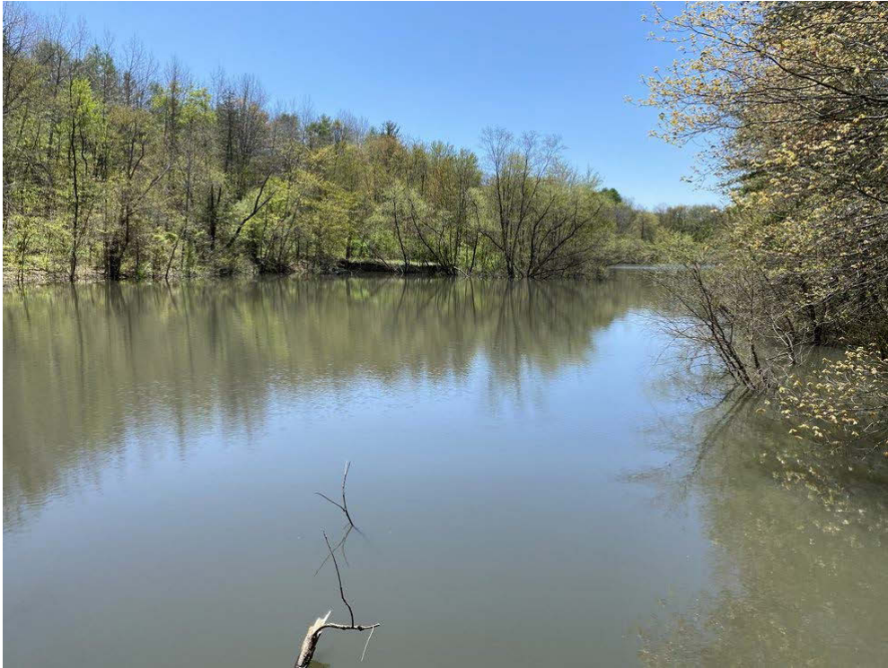
Figure 4-31: E41186777597290 "Leuders Creek Dam" standing on the dam looking west
