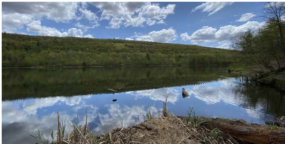
Figure 4-22: E41174187598896 “Hanover Reservoir” standing on dam looking southwest
