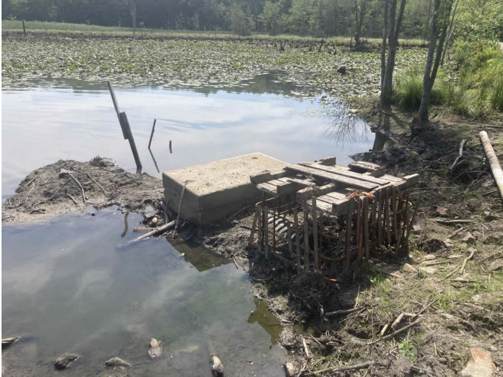
Figure 3-14: E41206457593751 "Hanover Crossings NBLT Wetlands (T)" looking southeast at outlet
