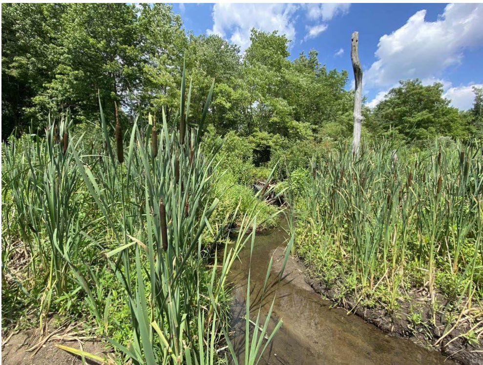
Figure 3-11: E41211367594534 "Below Hanover Crossing Road Culvert (M)" looking northeast
