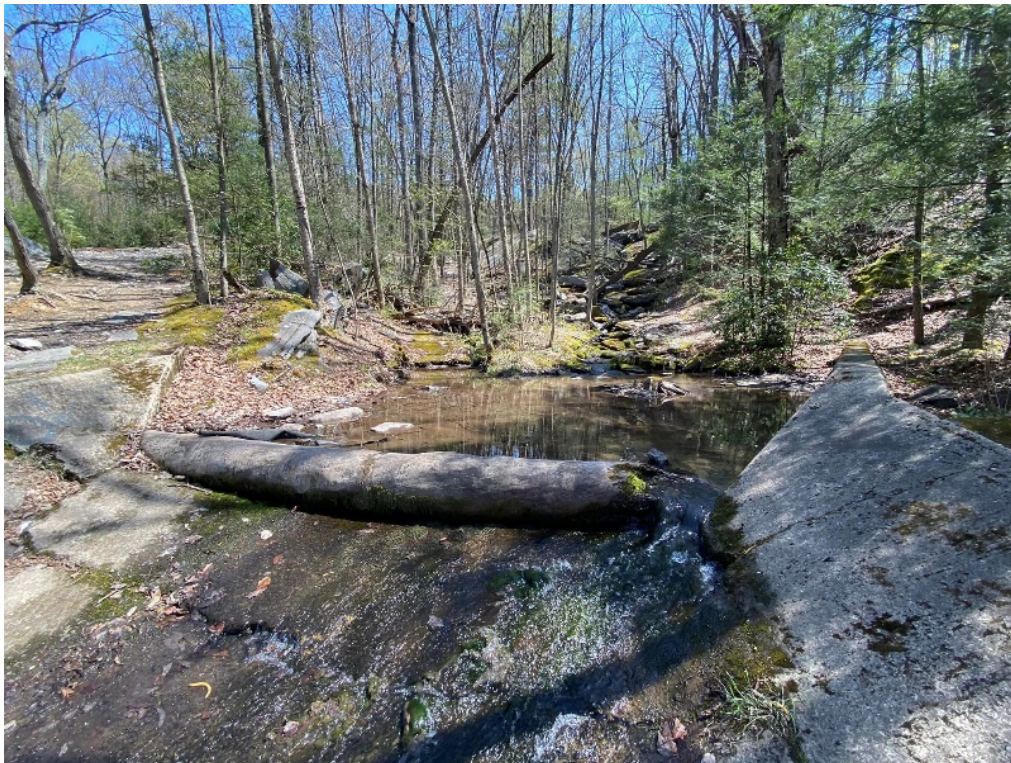
Figure 6. Headwaters of Nanticoke Creek upon entering the Concrete Flume
