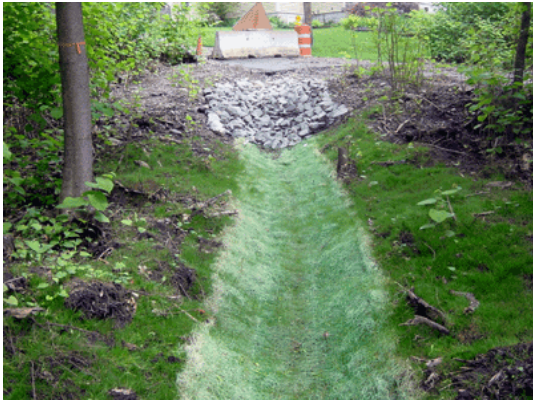
Figure 5. A vegetative swale using a sod base with a rock filter at the end of the swale.
