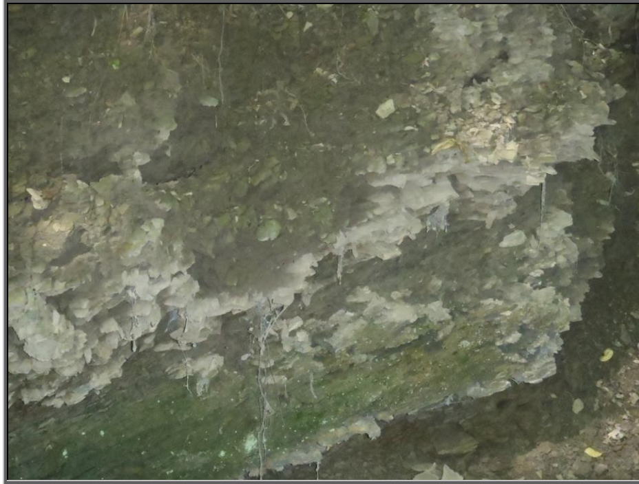
Photo : Shaley outcrop along the left streambank of Sugar Notch Run that was highly erodible and is the probable source of most of the shaley streambed further downstream before entering Carey's Patch
