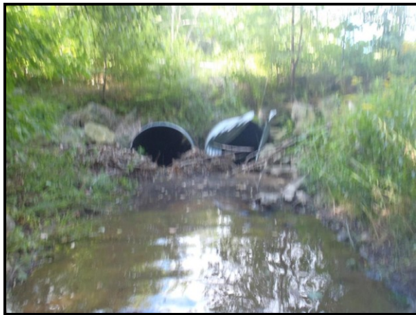
(L) Photo: Corrugated Steel double pipe culverts looking downstream on Sugar Notch on the other side of the entrance road to the Hanover Mini-Hawks Football practice area; Culverts are blocked up and could be cleared of debris with minimal effort
