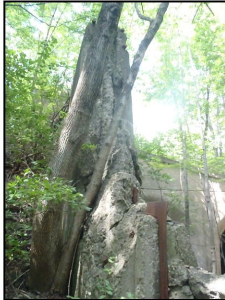
(L) Photo: Remnants of the old concrete dam with rebar exposed along the left stream bank looking upstream
