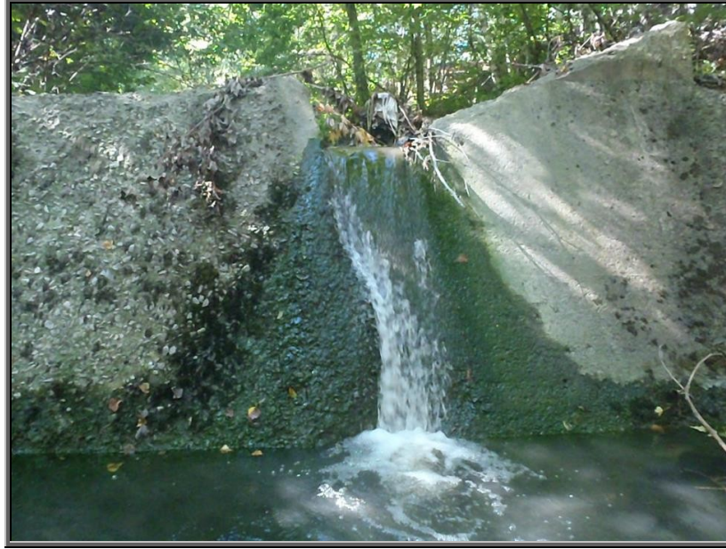
Photo : Close up of the overflow area at the concrete dam on Sugar Notch Run; This dam should be recommended to be removed to allow for potential fish passage from upstream areas down through Sugar Notch Run as a stream improvement and habitat restoration project
