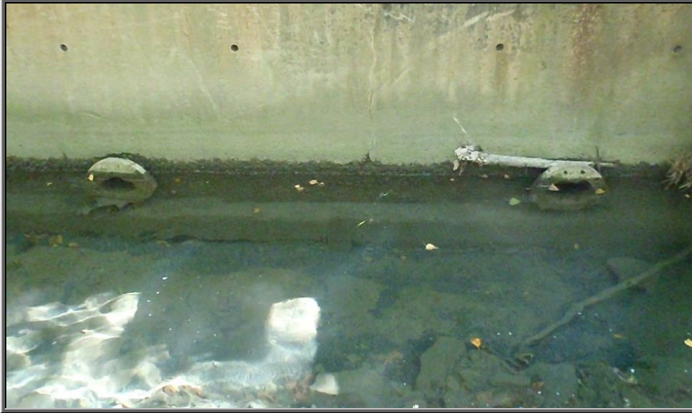
(L) Photo : Two intake pipes along the foundation wall of the abandoned Huber Breaker Colliery Pump House along Sugar Notch Run
