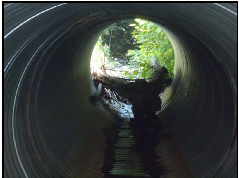
Photo: (L & R): The culvert pipe on the left is clear of any debris looking upstream and the culvert pipe on the right is blocked with a large tree and other woody debris; This culvert on the right is in need of a small debris removal project to remove the hazard to the road crossing into the Industrial Park and Hanover Township Youth and Recreation Center
