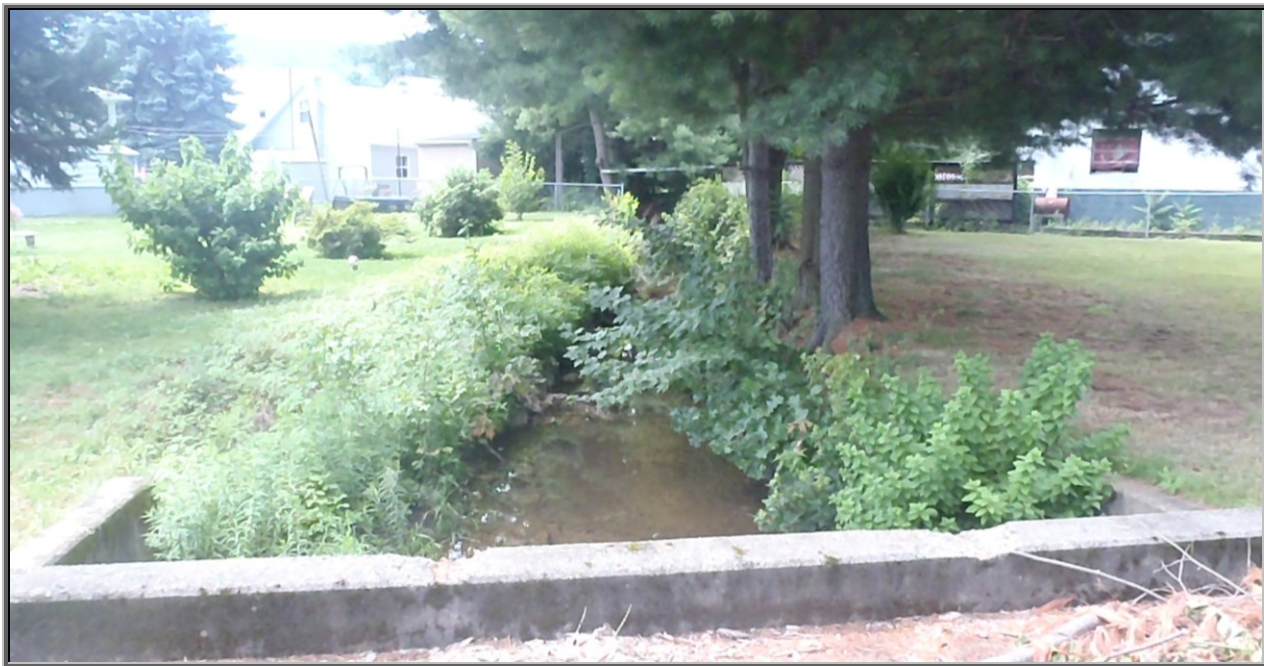
Photo : Sugar Notch Run flowing through Carey's Patch looking upstream through some private yards where the tributary has been modified and channelized heavily by residents probably to prevent further flooding incidents in their yards
