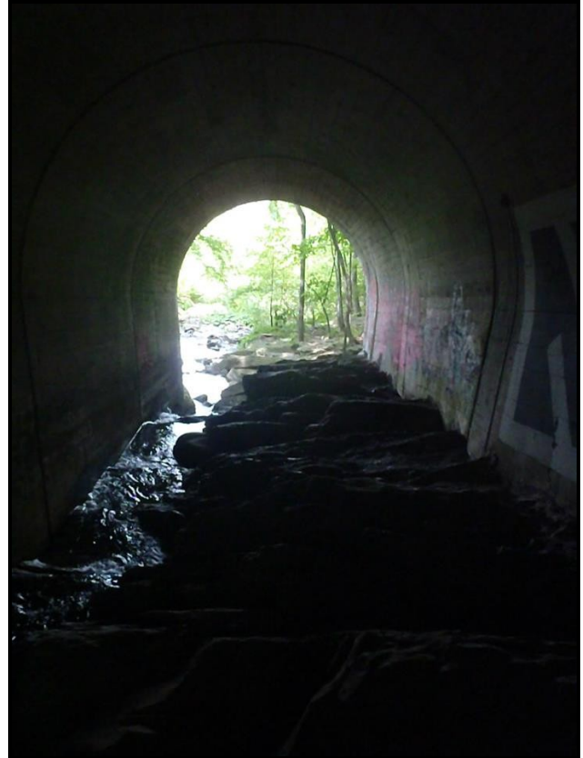
(L) Photo: Sugar Notch Run flowing through the newer constructed tunnel underpass looking upstream; Notice the bedding planes are steeply pitched and faulted
