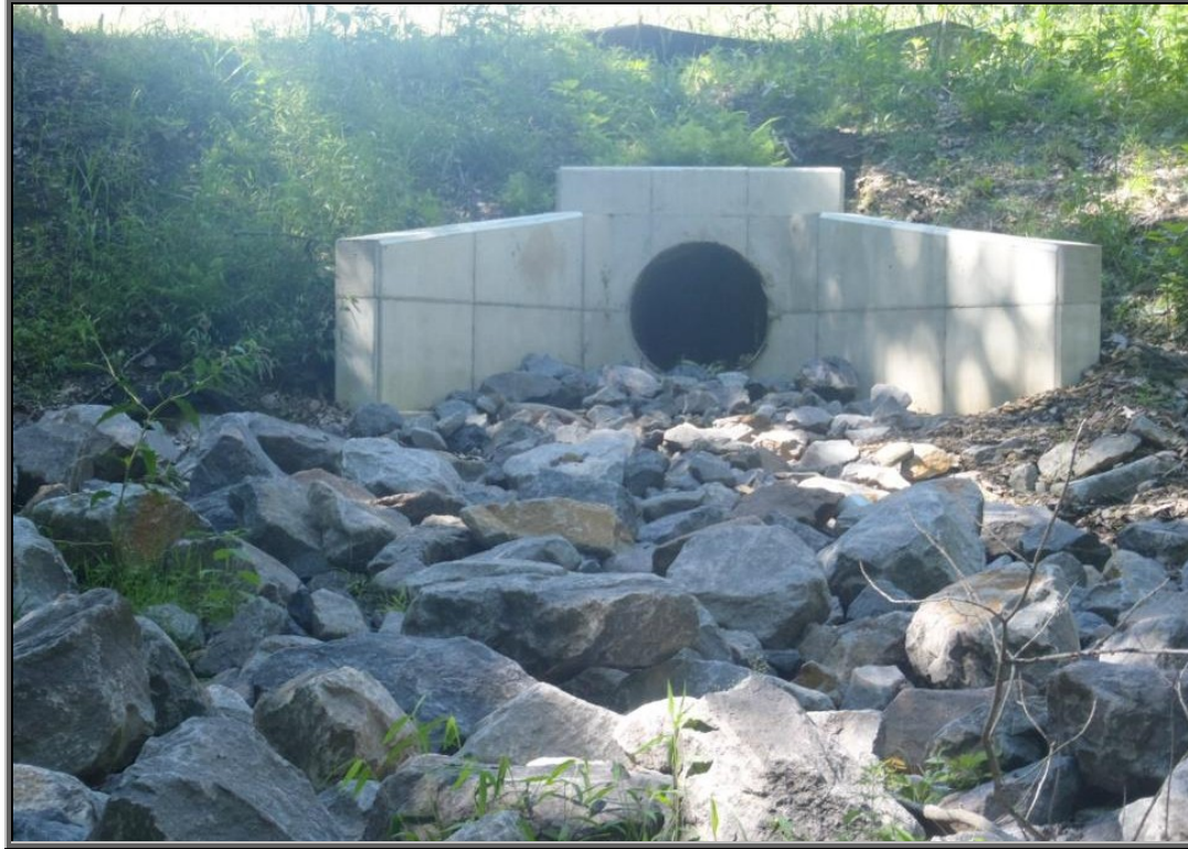
Photo : Stormwater culvert or ephemeral unnamed tributary to Sugar Notch Run with rock apron on the left streambank coming off the Huber IV AML Reclamation Site completed by the Earth Conservancy
