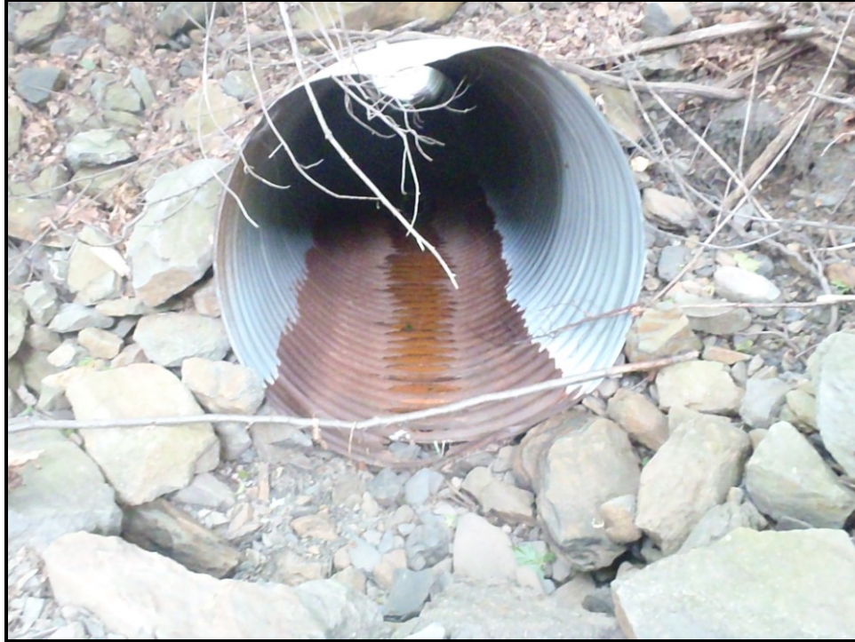
Photo : Looking downstream on what would be Sugar Notch Run, if it were flowing into the drainage pipe; In this location it is a losing reach through the porous culm, rock, and shale in the area
