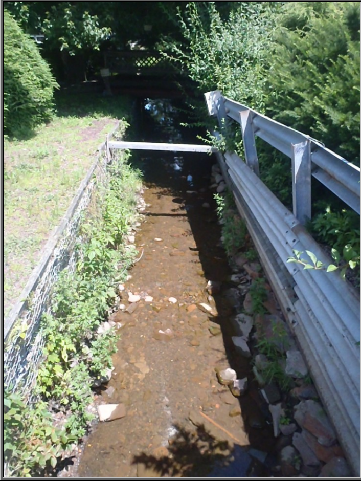
Photo : Sugar Notch Run looking downstream from the other end of Carey's Patch through some private yards where the tributary has been modified and channelized heavily by residents probably to prevent further flooding incidents in their yards using gabion baskets and guiderrails
