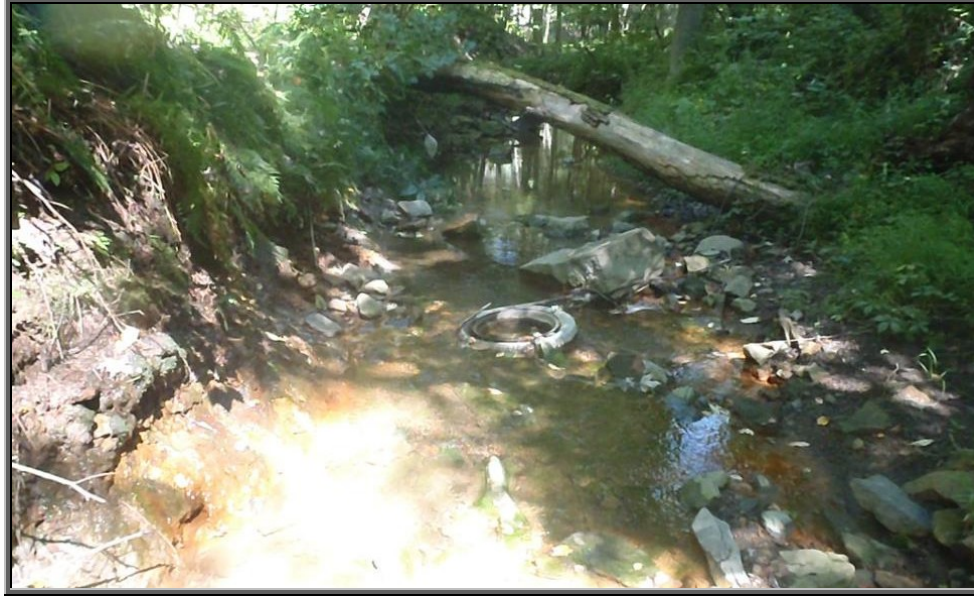
Photo : Presence of iron hydroxide becomes readily apparent within Sugar Notch Run within 100' downstream of the railroad tunnel from within the streambed itself with no apparent discharge locations in sight; Debris is littered throughout this reach
