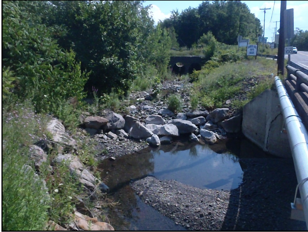
Photo : Gravel bar deposition, point bars, and a check dam of sorts along the upstream side of the bridge over S. Main Street as Sugar Notch Run continue up upstream towards Preston Road; Removal of the gravel and point bars are recommended to prevent future flooding situations from occurring along S. Main Street
