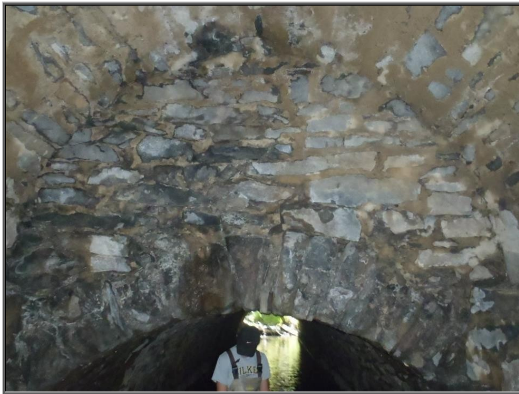
Photo: A second grouting of the original section of the railroad tunnel; Interesting mason work and keystone work on the arch; Justyna making her way through Sugar Notch Run and the tunnel looking upstream back towards the Preston section of Ashley Borough
