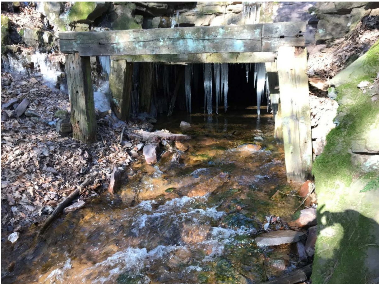
Figure 6. The Green Mountain Tunnel Outfall into Catawissa Creek
