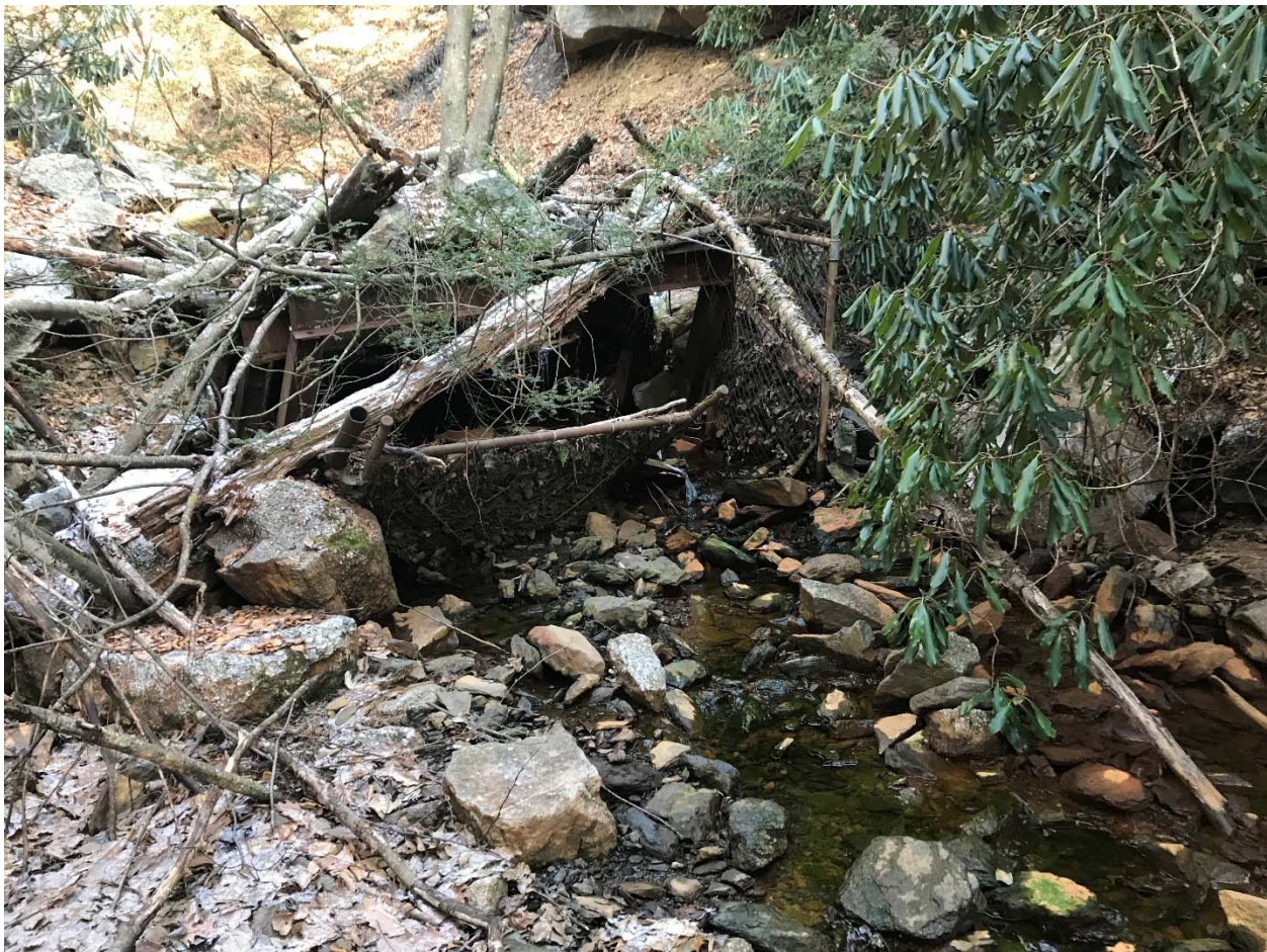
Figure 10. The Catawissa Tunnel Outfall into Catawissa Creek
