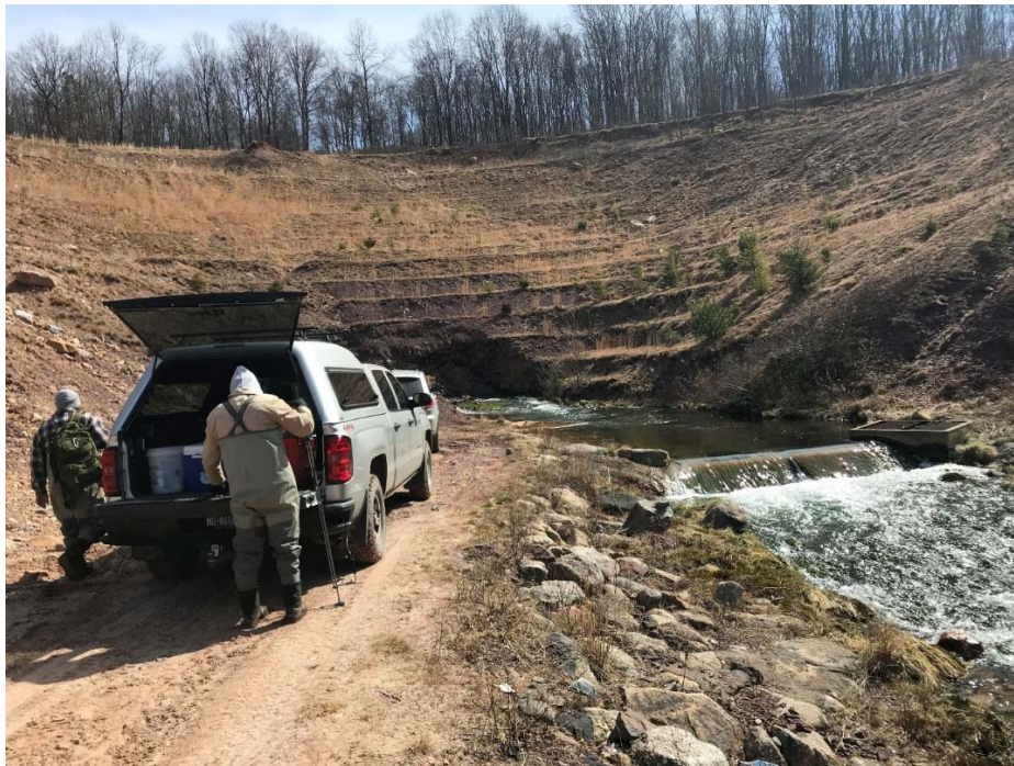
Figure 2. The Audenried Tunnel Outfall into Catawissa Creek
