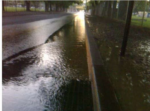
Woodward Colliery borehole (near Kirby Park) discharges into the storm drains when the river level is high.
