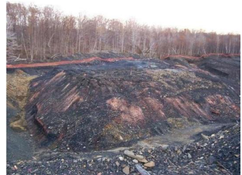
Trenches dug to help extinguish the Dolph Mine Fire near Olyphant, PA that has been burning for approximately 3 years now.
