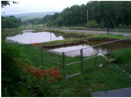
Fence installed around the SCRA Site 15 Treatment System along Rte 901 near Ranshaw, PA
