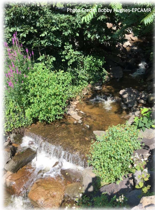
Figure 9. Wildcat Falls, unnamed tributary to Toby Creek flowing over concrete encased sewer line
