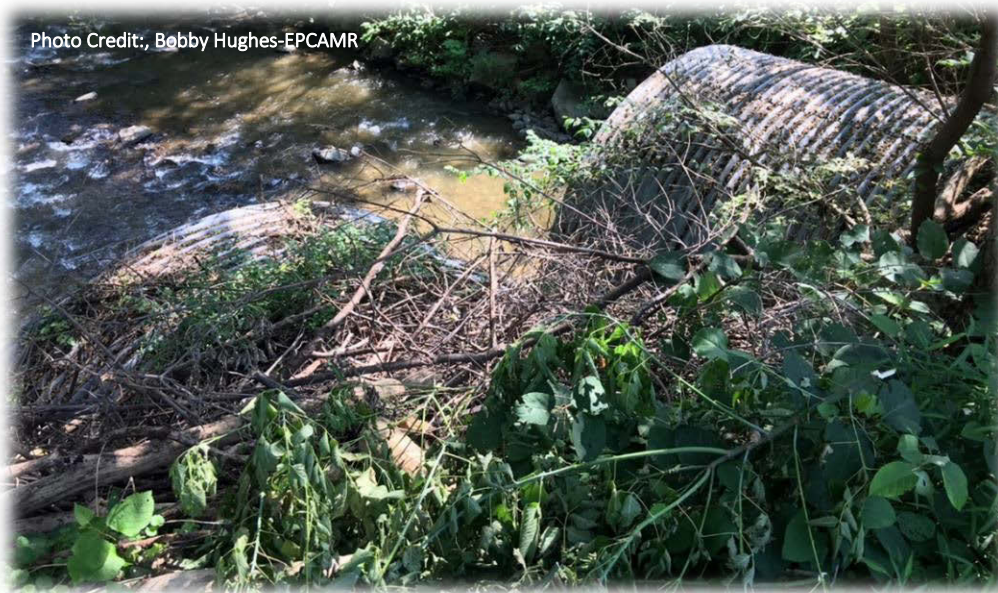
Figure 11. Double Metal Corrugated Squashed Pipes directing flow of Toby Creek under State Route 309 adjacent to the DAMA
