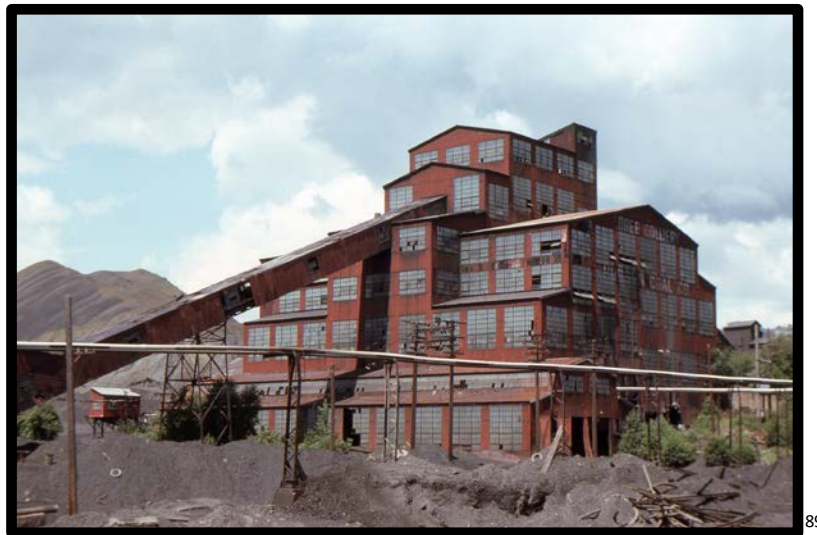
Figure 48. Loree Colliery Breaker
