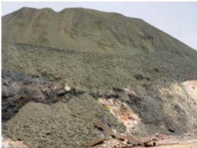
The 40-ft high Harry E. Breaker Waste Coal Pile, which was on fire, continues to be a source of pollution in Swoyersville, PA.
