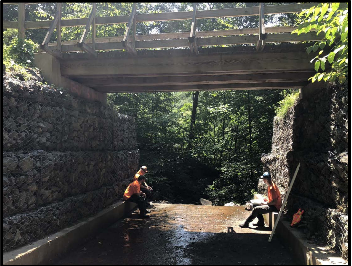
Figure 56. EPCAMR staff and partners beneath bridge above Wildcat Falls conducting a culvert assessment
