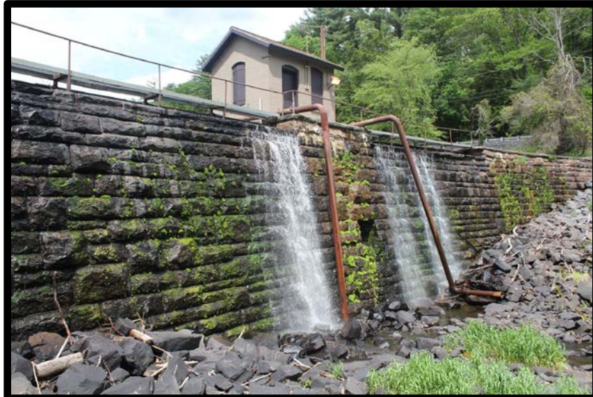
Figure 5. Present view of Huntsville Dam; Photo credit: Levi Sunday-Lefkowitz - EPCAMR
