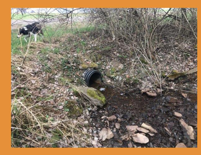
View of HDPE pipe on other side of cart path that receives the pump used in the pond in Fig. 17-18
