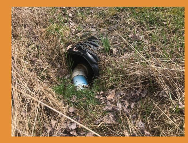
View of drop-in culvert that carries flow from wetlands in Fig. 20-21 further toward Rte. 115
