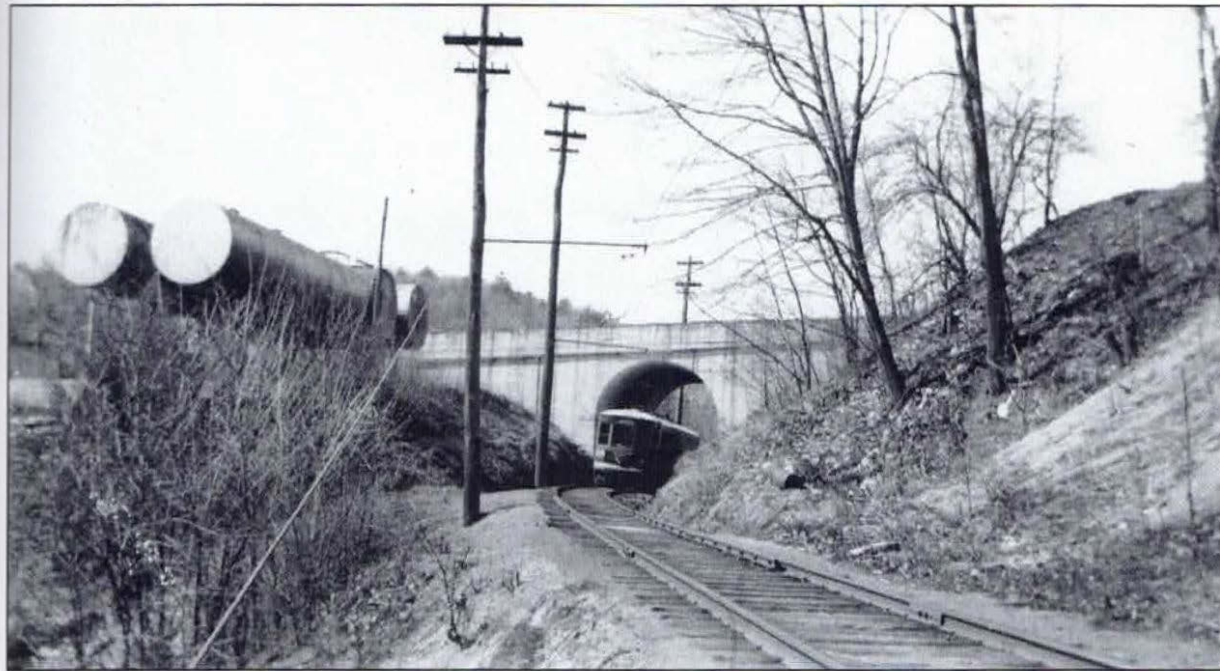
WILKES-BARRE RAILWAY CORPORATION TROLLEY NO. 332, MARCH 25, 1938. This photograph shows the underpass of the Harris Hill Road concrete bridge after the stone bridge was rebuilt and the second arch was removed. Toby's Creek was diverted through the arch after trolley service was discontinued and the trolley tracks were removed. (Courtesy of the Edward S. Miller collection.)
