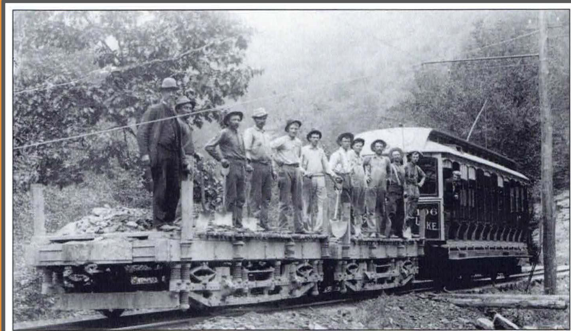
FOREMAN EDWARD BAER AND WORKMEN, c. 1897-1898. The men are pictured on a flatbed and trolley No. 106 near the Harvey's Lake trolley station. The trolley line was built by the Wilkes-Barre, Dallas and Harvey's Lake Railway Company to attract tourists to Harvey's Lake. Several stockholders in the company incorporated the Harvey's Lake Hotel and Land Company to construct the Oneonta Hotel on April 20, 1897. (Courtesy of the Misericordia University Archives.)
