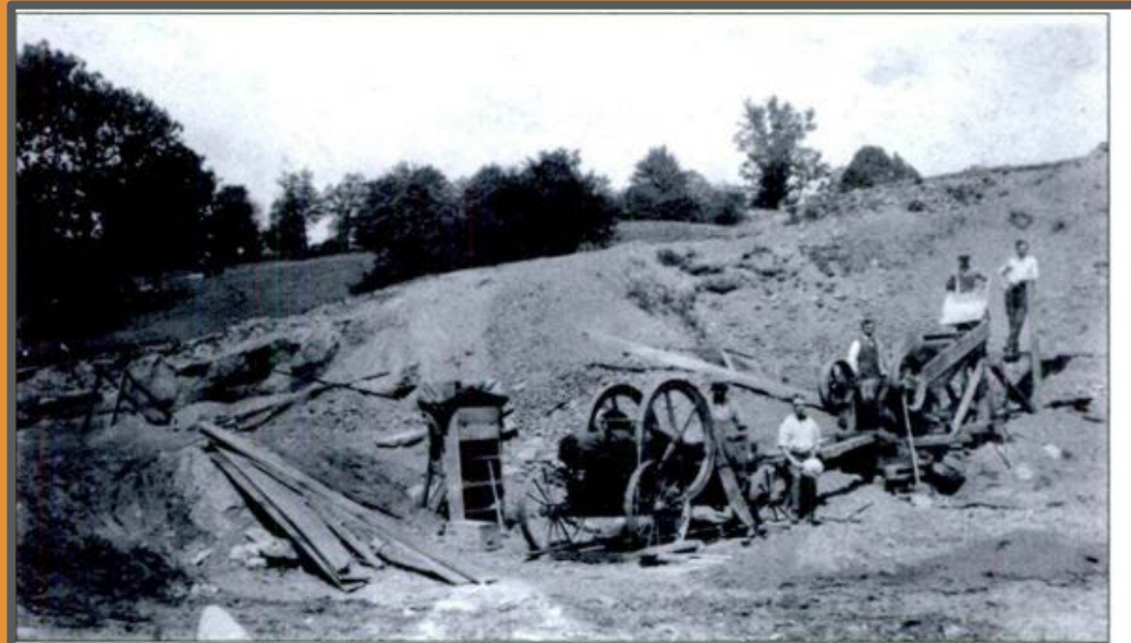
SAND AND GRAVEL QUARRY, c. 1898. The quarry was located near Sutton Road on the farm owned by Wesley David Sutton (1862–1942), pictured in the center. Sutton Road was laid out in 1803 between the Fuller and Baldwin mills bordering property owned by William Trucks. The quarry overlooked Hillside Farms. Hillside Farms purchased the Sutton farm from the estate of Wesley David Sutton in 1946. (Courtesy of Joan Coolbaugh Britt.)
