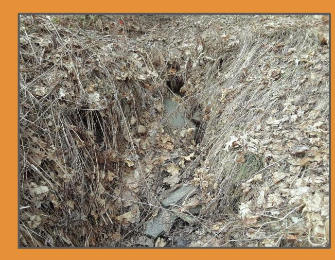
Upstream view of same HDPE pipe in Fig. 10 on the other side of the small road in the golf course. Half full of sediment and leafy debris
