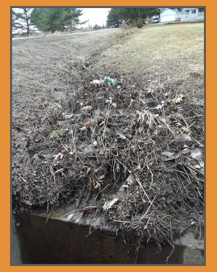
View of square stone drop-off that holds groundwater and flow from pipe in Fig. 13. Flow drains through larger HDPE pipe to other side of small road on the golf course.
