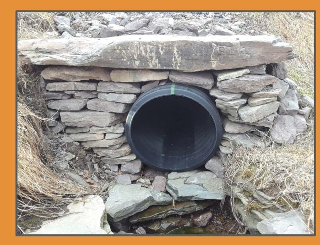
Upstream view of HDPE pipe from Fig. 14 that crosses road in the golf course. A small amount of sediment in pipe.
