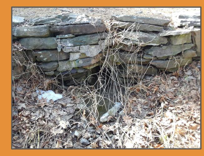
2 12" concrete pipes in square drop-off that pass under Huntsville-Idetown Rd. - Half full of leafy debris and sediment
