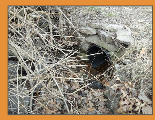
Upstream view of opposite side of culvert under Old Rte. 115. -Completely blocked with debris and leaf litter.
