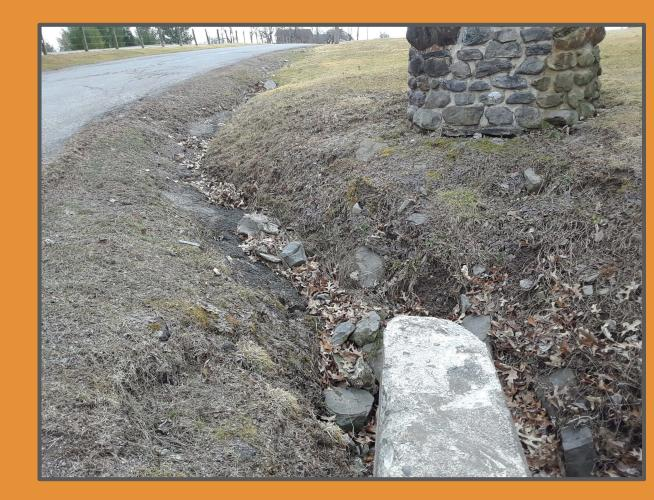
Downstream view of Fig. 3. 18-inch HDPE culvert that passes under Hayfield Rd. - Some leaf matter, small white pipe from adjacent property
