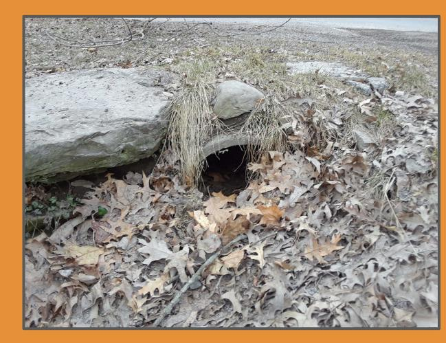
Downstream view of rectangular culvert with 18-inch HDPE pipe, mortared into larger concrete pipe with rocks.
