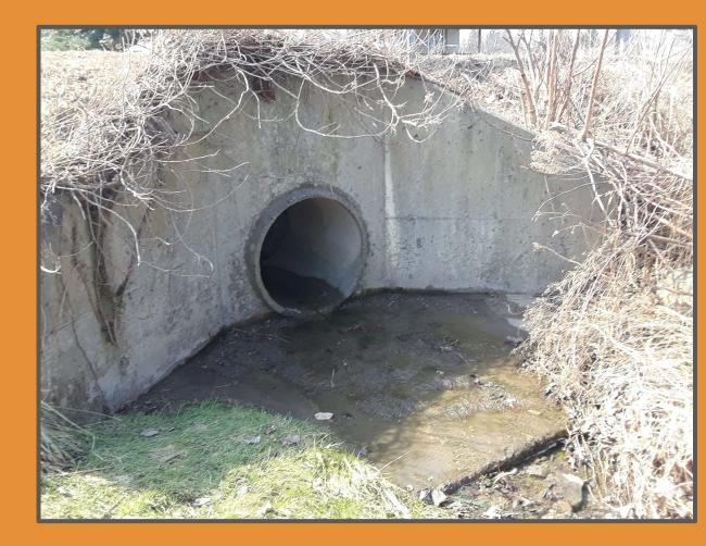
Upstream view of 30-inch corrugated metal pipe bringing drainage from Lake Lehman Early Learning Center. Pipe is corroded along base of the structure.
