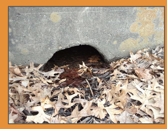
Upstream view of flow from culvert in Fig. 20 on the other side of Old Rte. 115. Full of leaf litter that is clogging the pipe.
