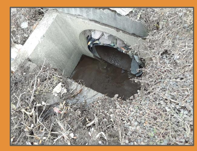
Upstream view of same drainage from Fig. 6. It drops to a rectangular concrete culvert with an 18-inch HDPE pipe, receives flow from both Old Rte. 115 and Market St., then passes under Old Rte. 115 to the Huntsville Golf Course.
