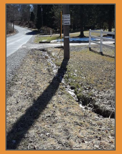
Downstream view of UNT in Fig. 86 flowing into 18" concrete pipe under stone headwall as it crosses under Huntsville-Idetown Rd.
