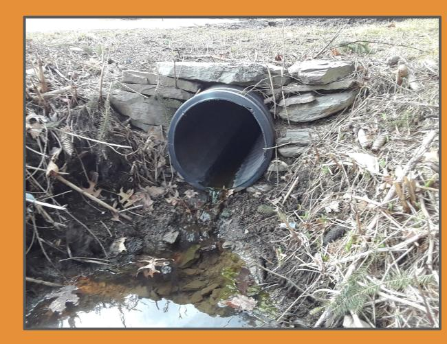
Downstream (DS) view of culvert from Fig.1. 18-inch with some rocks and debris blocking drainage
