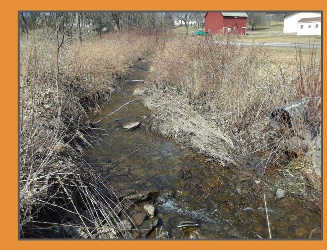
View of 2-3' metal pipe carrying UNT under Goodman Rd. Pipe has some build up of sediment, but flow is level through the pipe relative to the UNT
