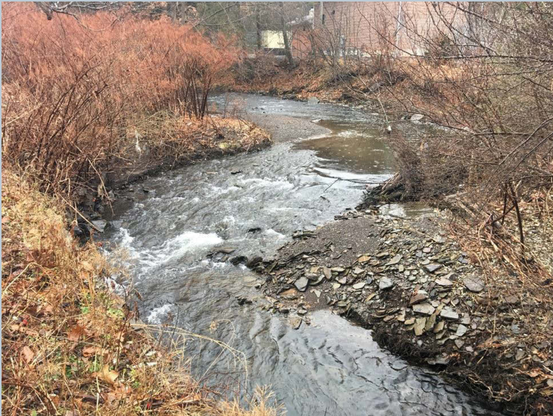
Figure 149. In this section of Toby Creek, there is severe undercutting of the streambank along N. Main Street and the opposite bank, alongside a utility shed. This is due to the 90-degree turn into the right bank, while looking upstream. A streambank stabilization project is recommended.
