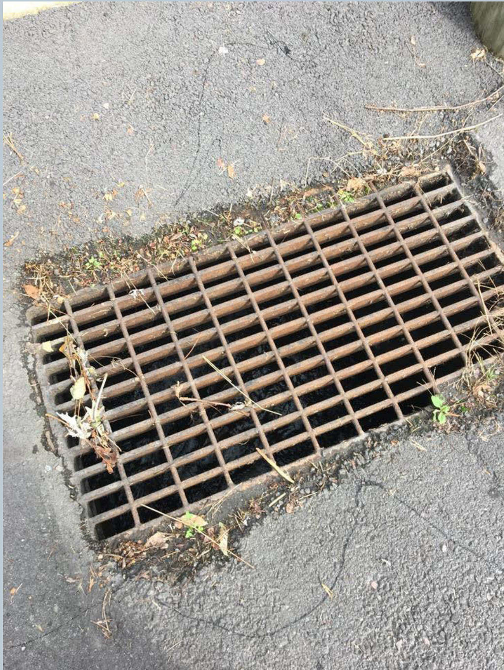
Figure 61. An outlet of storm drain from the unnamed tributary to Toby Creek at the intersection of W. Center Street and N. Pioneer Avenue.
