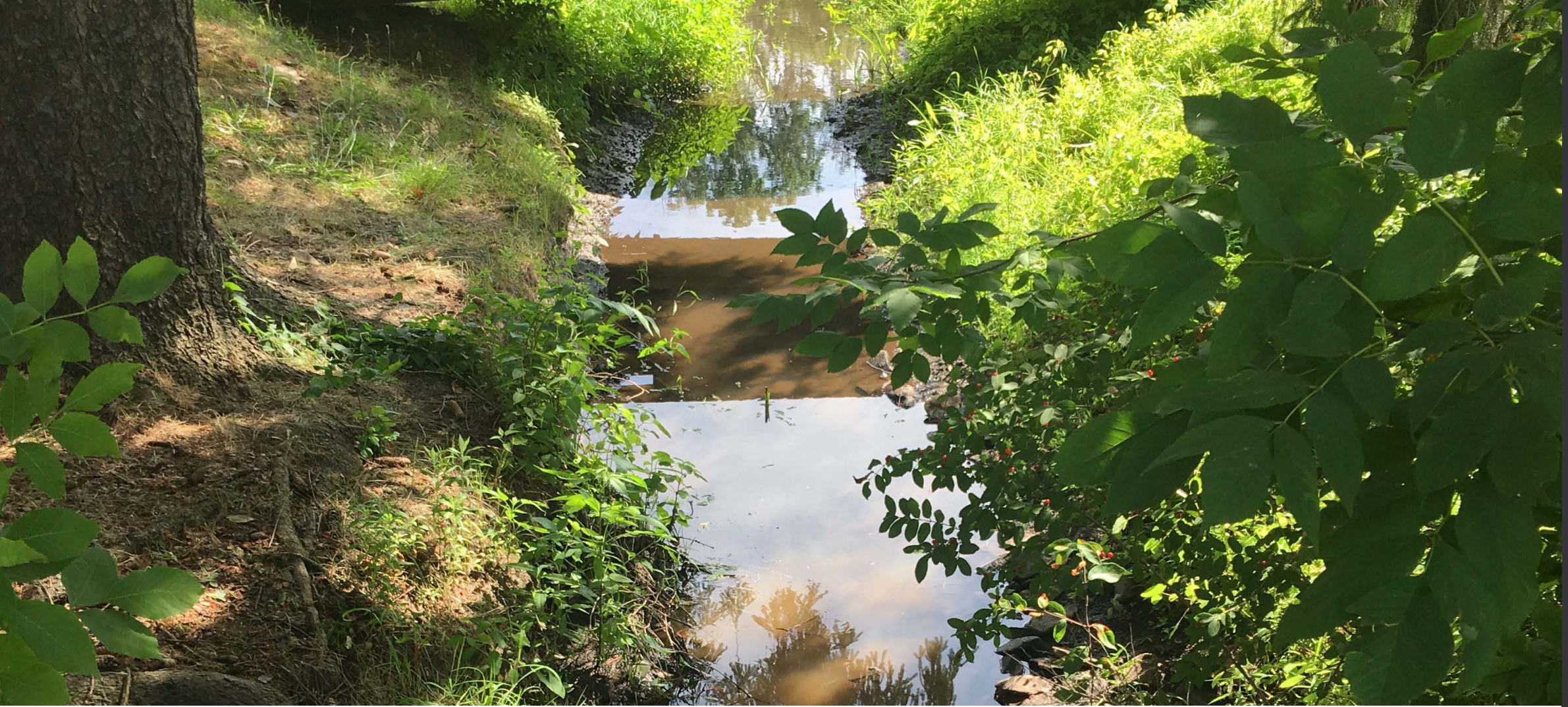
Figure 194. Upstream of Inlet pipe at the dip in Irem Road at the bottom of the hill. Catfish were present. A severe constriction exists upstream. Pipe is recommended to be replaced to a larger box culvert. A small riparian restoration could be implemented in this area.
