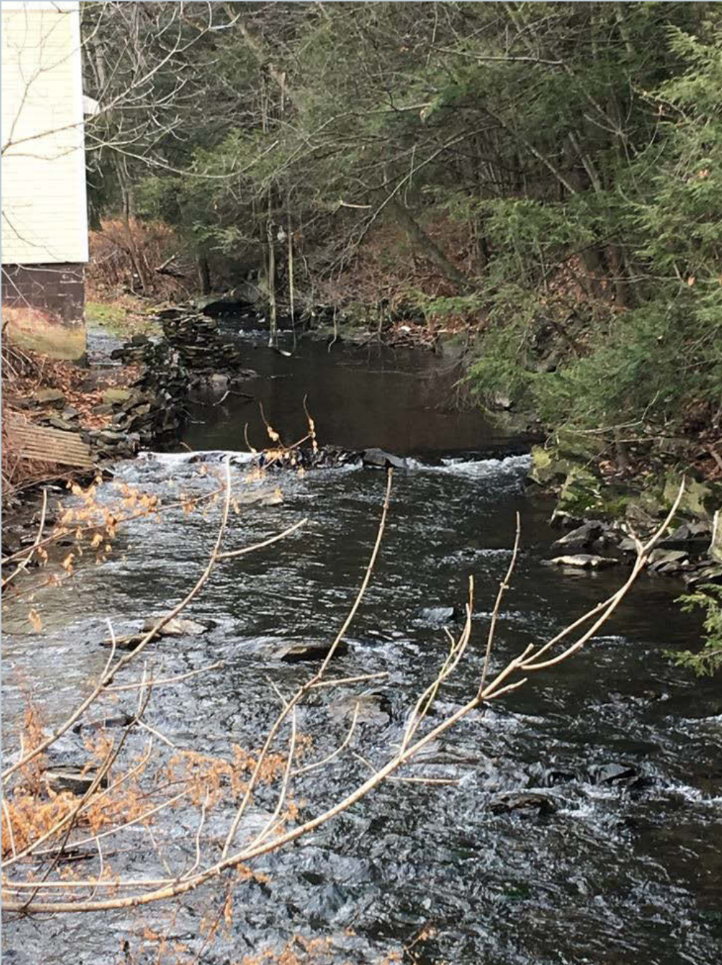
Figure 113. Behind Modern the Floor Store, a small dam is in Toby Creek which is creating a small pool.
