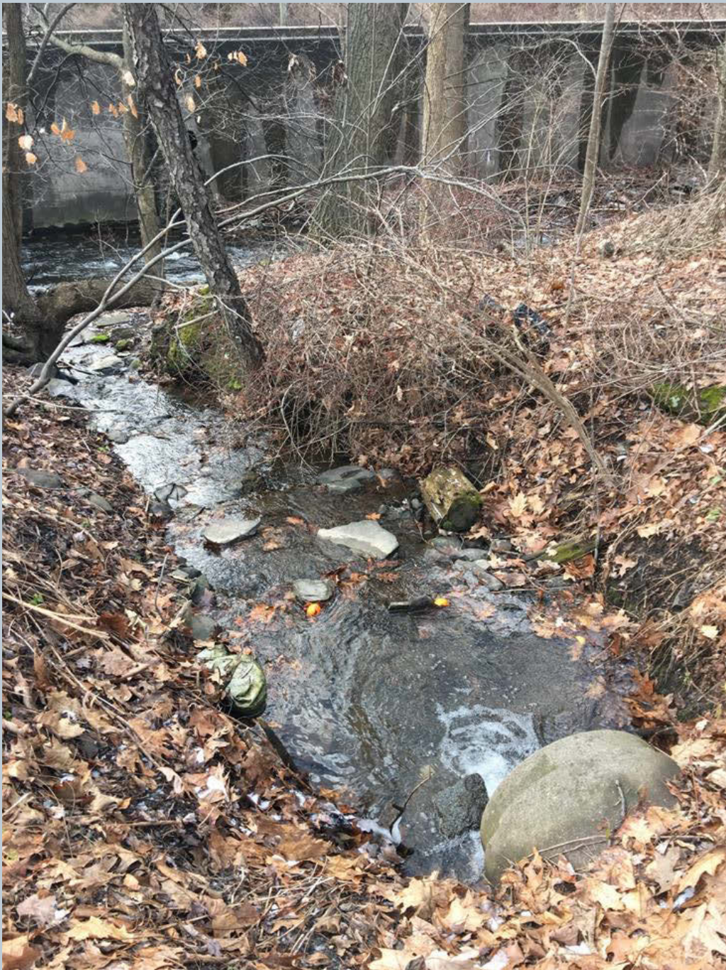
Figure 118. An UNT to Toby Creek flows from an 18-inch concrete pipe along N. Main Street and Division Street, which is aligned with Toby Creek.
