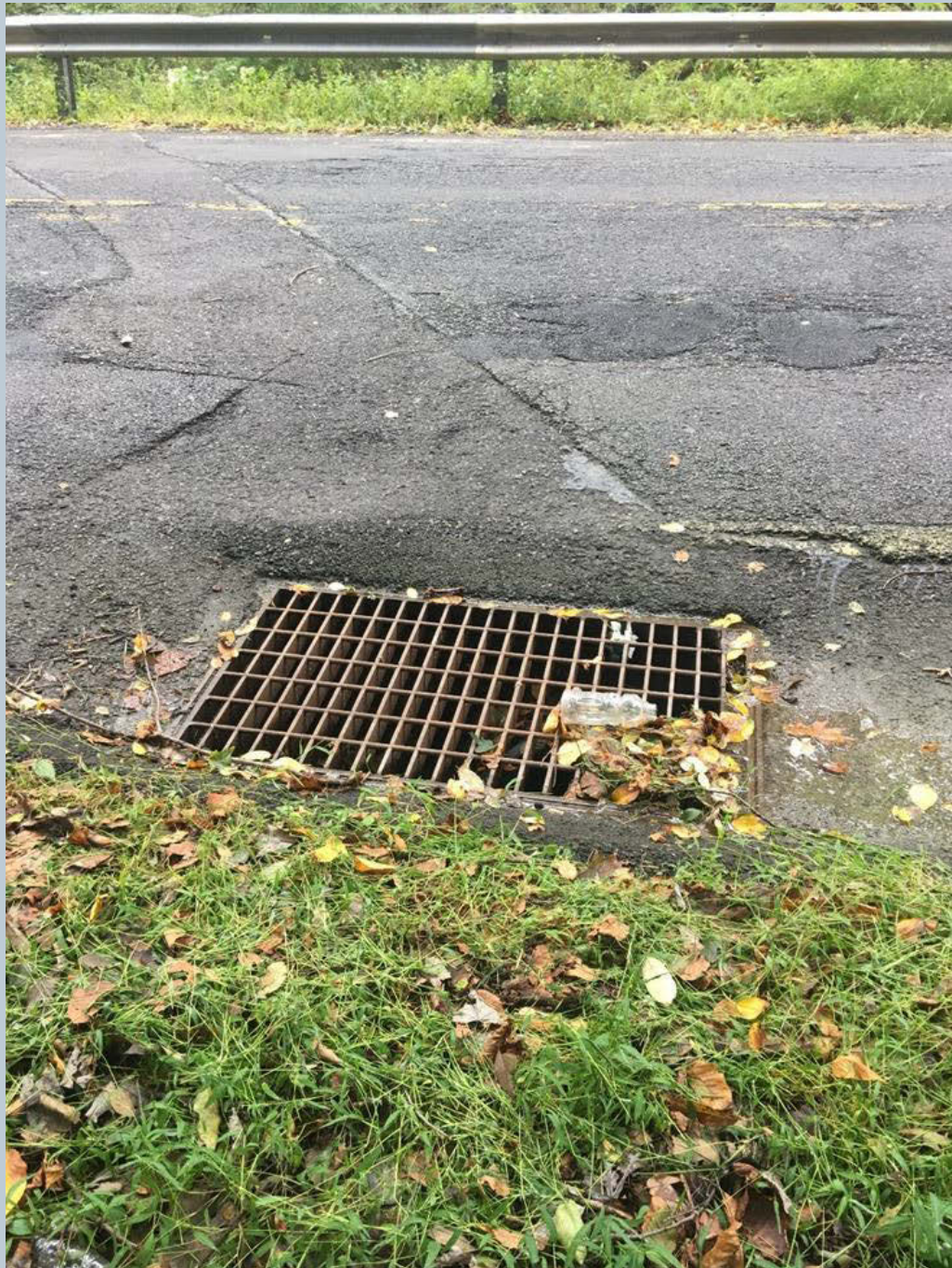
Figure 21. An 18-inch black HDPE stormwater pipe crossing Harris Hill Road.
