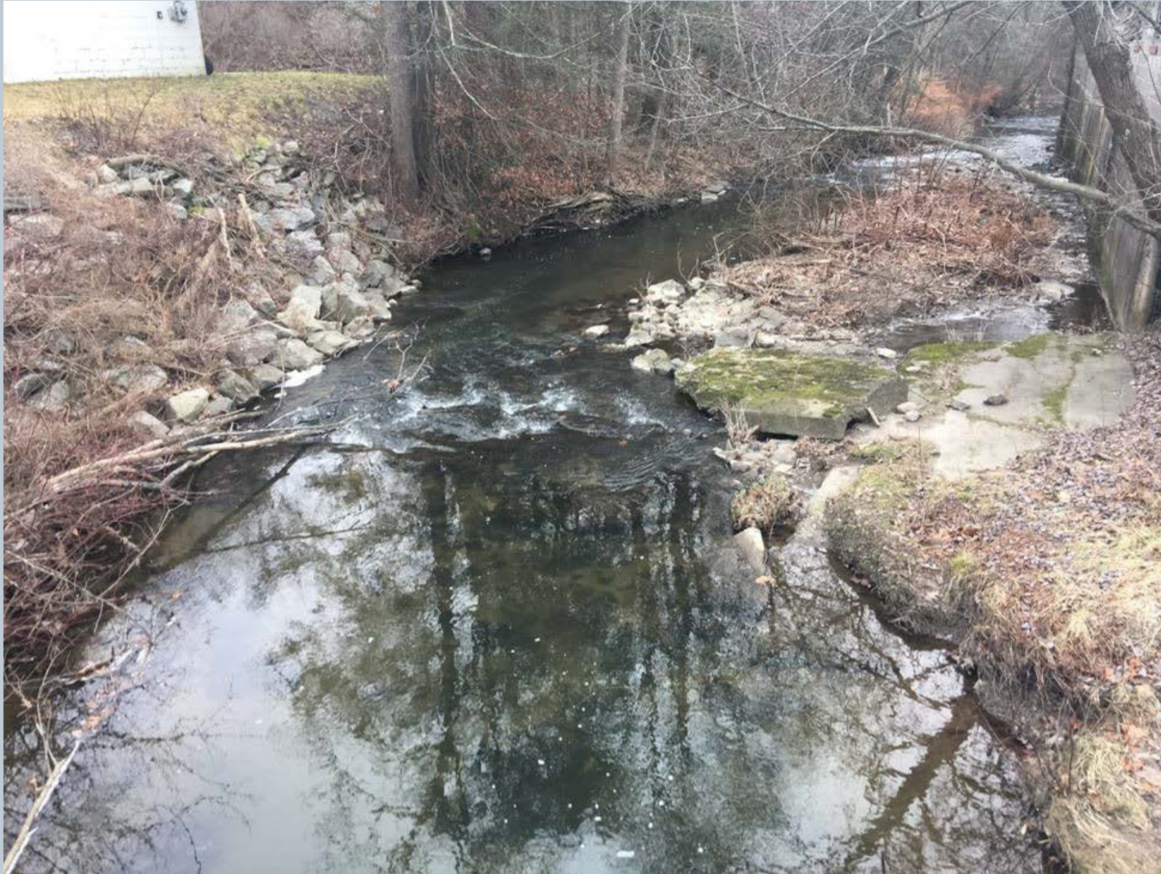
Figure 75. Looking downstream on Toby Creek from behind the Pen Fern Oil Gas Station from the bridge over Lower Demunds Road. A large historic rock stabilization placement is seen along the left bank while looking downstream, and there is bed rock present looking to the right of the stream. This bed rock is found adjacent to the Pen Fern Oil Gas Station's foundation that runs up against the right bank of Trout Brook.
