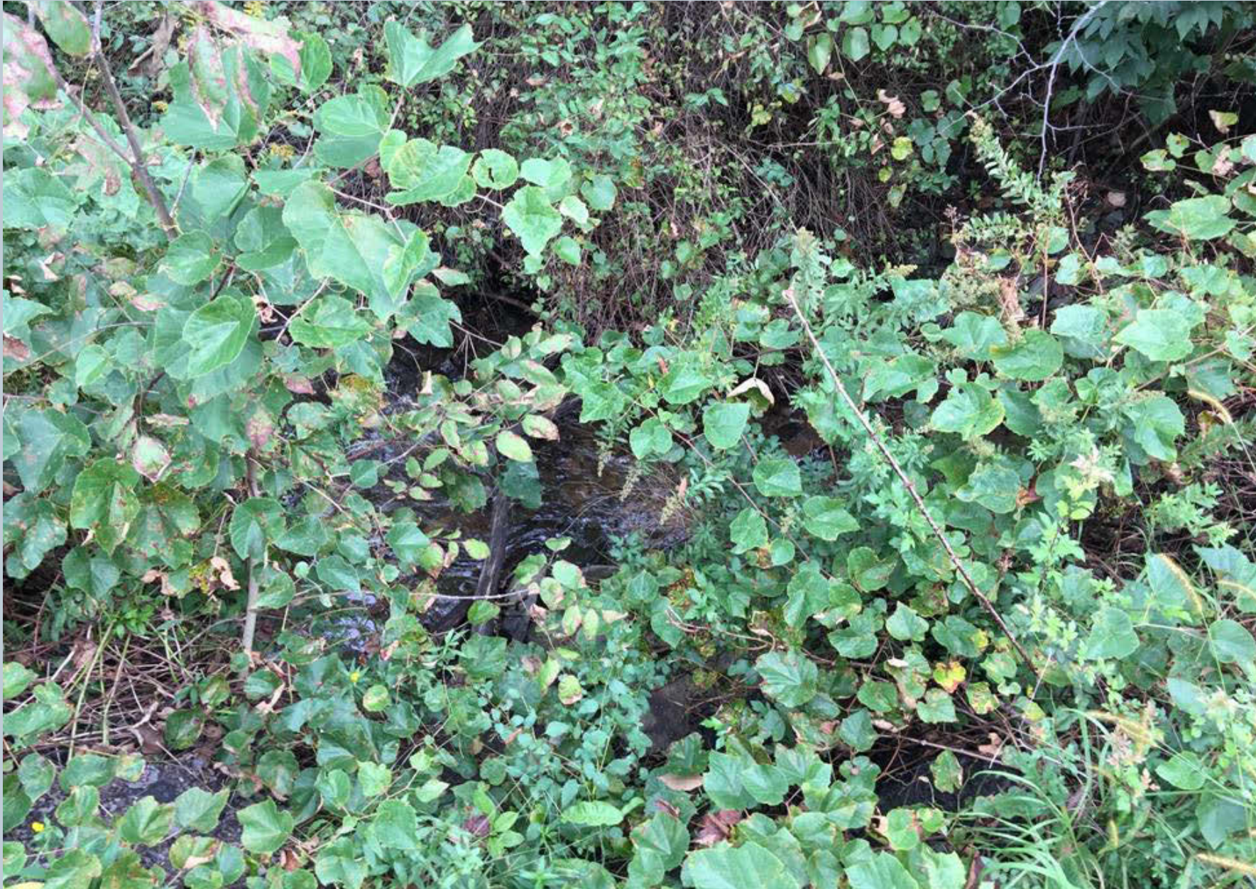
Figure 37. A box culvert on the Green Pond unnamed tributary, looking upstream.
