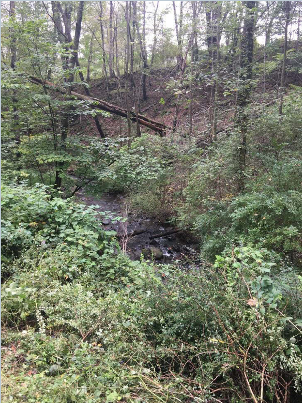
Figure 22. An 18-inch black HDPE stormwater pipe that outlets to the Green Pond unnamed tributary is present at this location. Invasive removal of Japanese barberry and Multi-flora roses is recommended.
