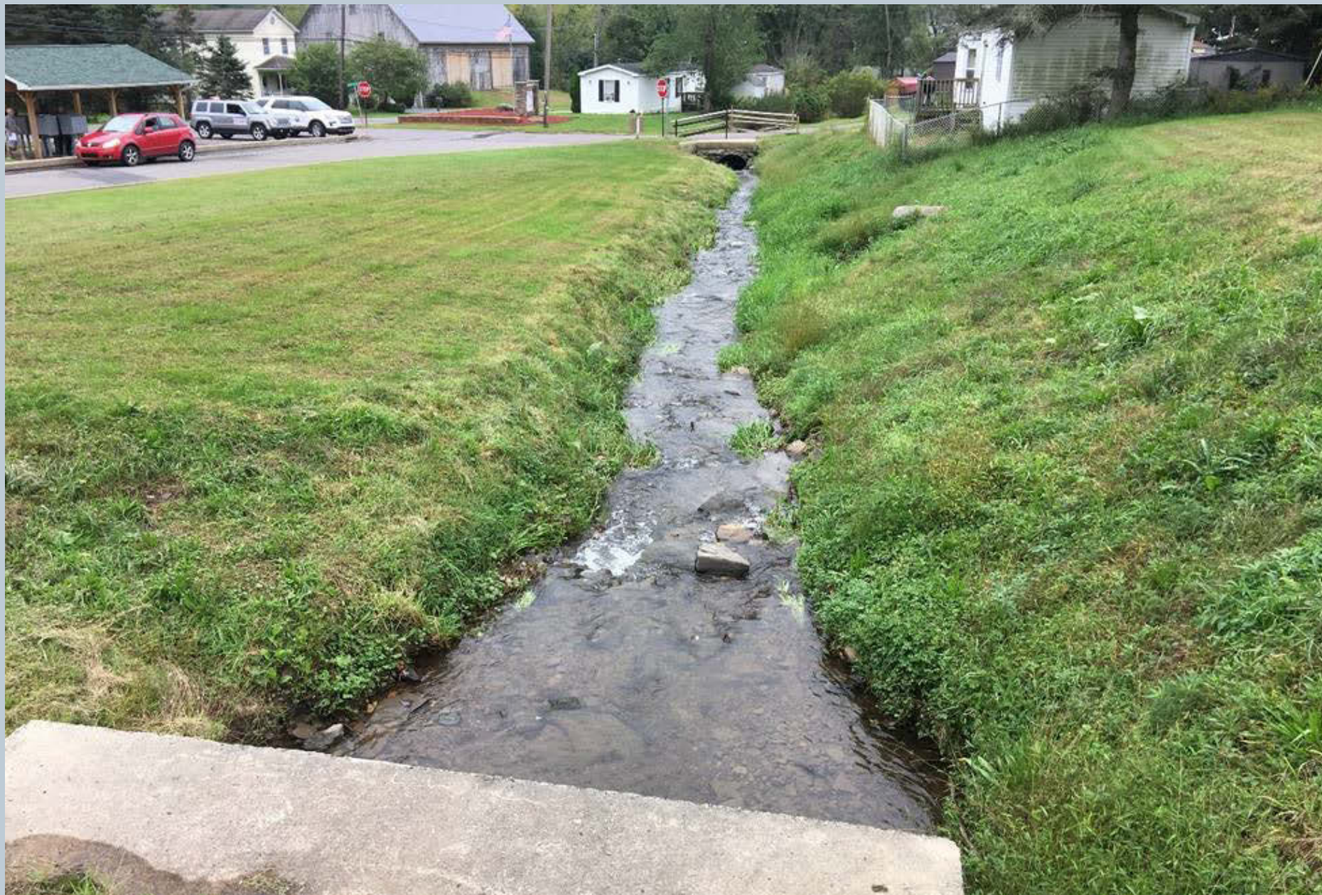
Figure 38. A box culvert on the Green Pond unnamed tributary, looking downstream.
