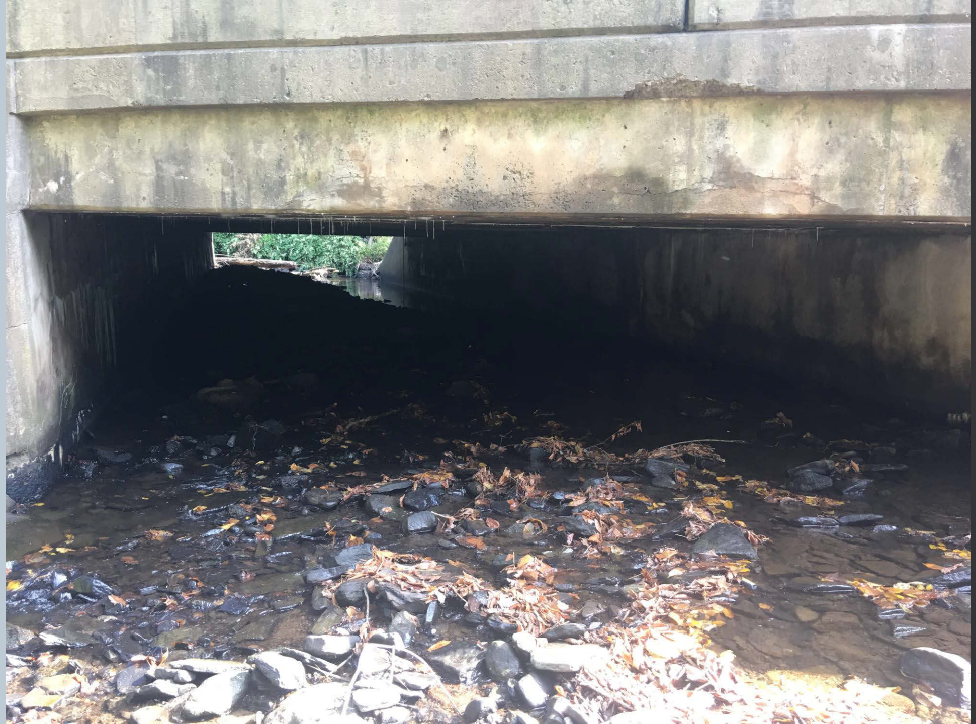
Figure 362. Looking upstream on Toby Creek near Modern Floors Professional Building from the outlet of one of the structures from the bridge culvert over the Dallas Memorial Highway where the majority of the flow can be seen and a gravel bar deposition at the inlet side of the structure of the culvert. Fish present.
