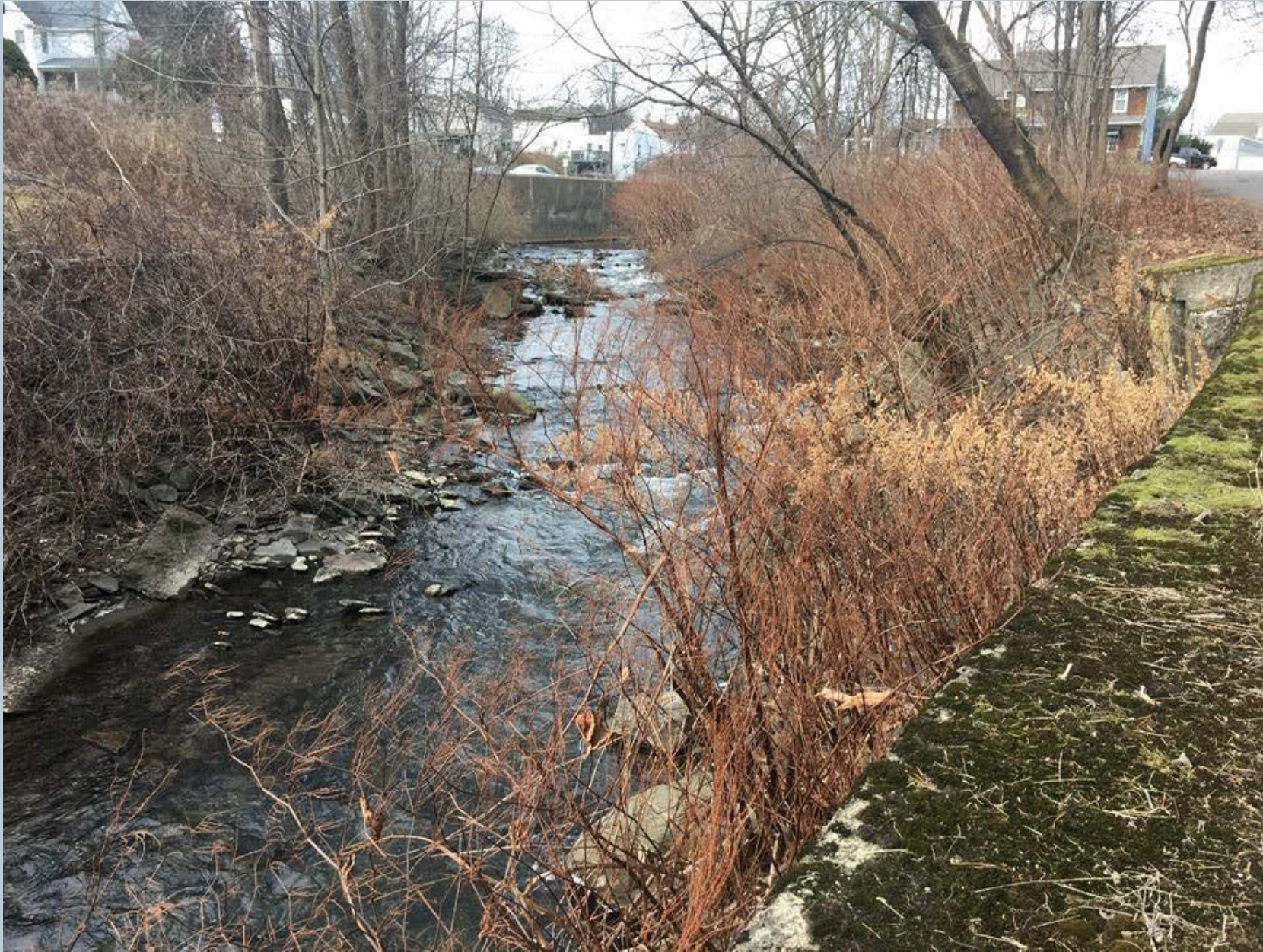
Figure 89. A shot looking upstream at Toby Creek from curved concrete retaining wall located along N. Main Avenue. Oriented in the direction of the Lonn Dean Salon and the North Memorial Highway concrete retaining wall, the presence of Japanese knotweed, an invasive, and a gravel bar deposition, opposite the retaining wall, on the inside of the bend of Toby Creek are present.
