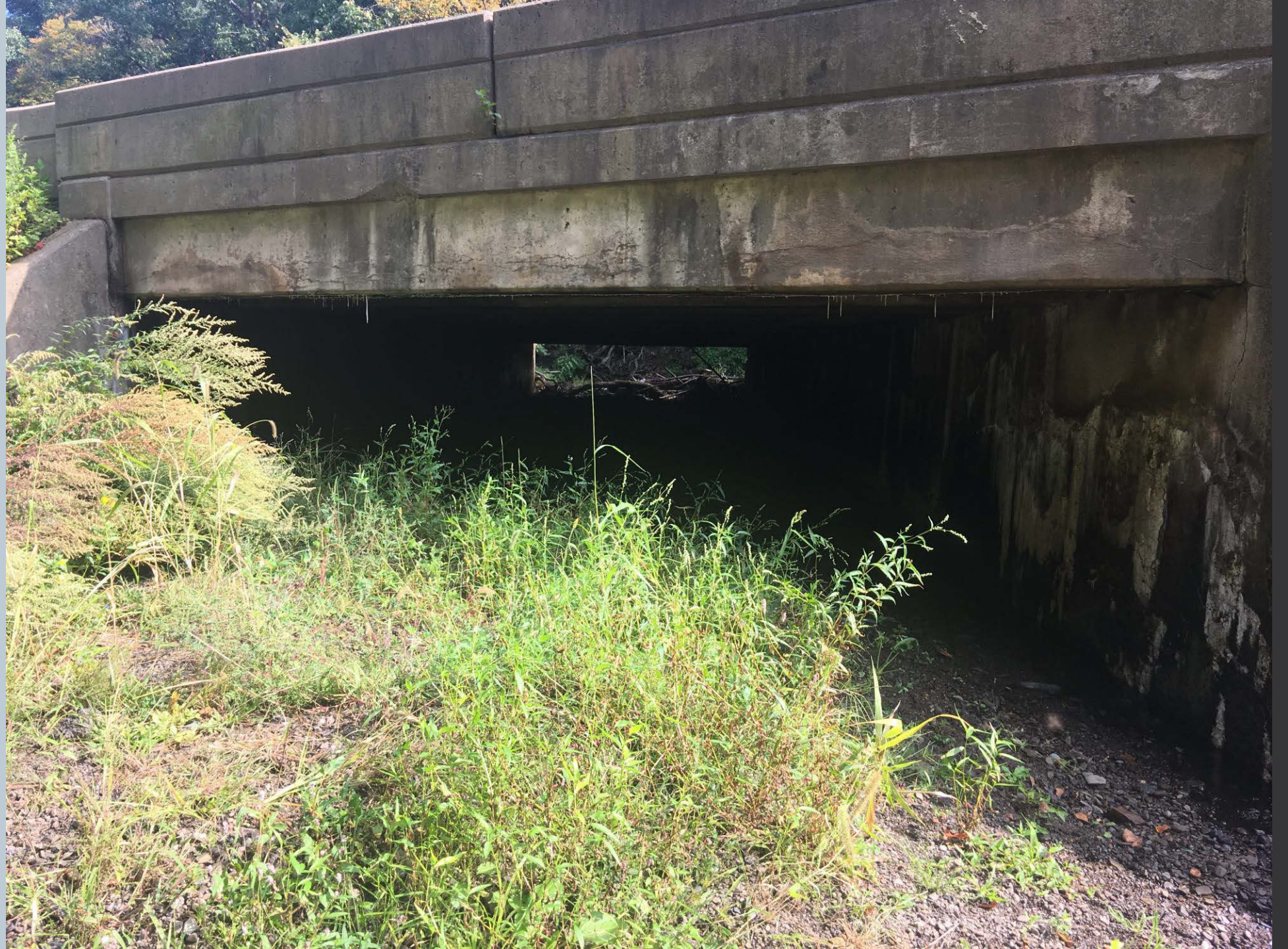
Figure 363. Looking upstream on Toby Creek near Modern Floors Professional Building from the outlet of one of the structures from the bridge culvert over the Dallas Memorial Highway where a gravel bar deposition at the outlet side of the structure of the culvert.
