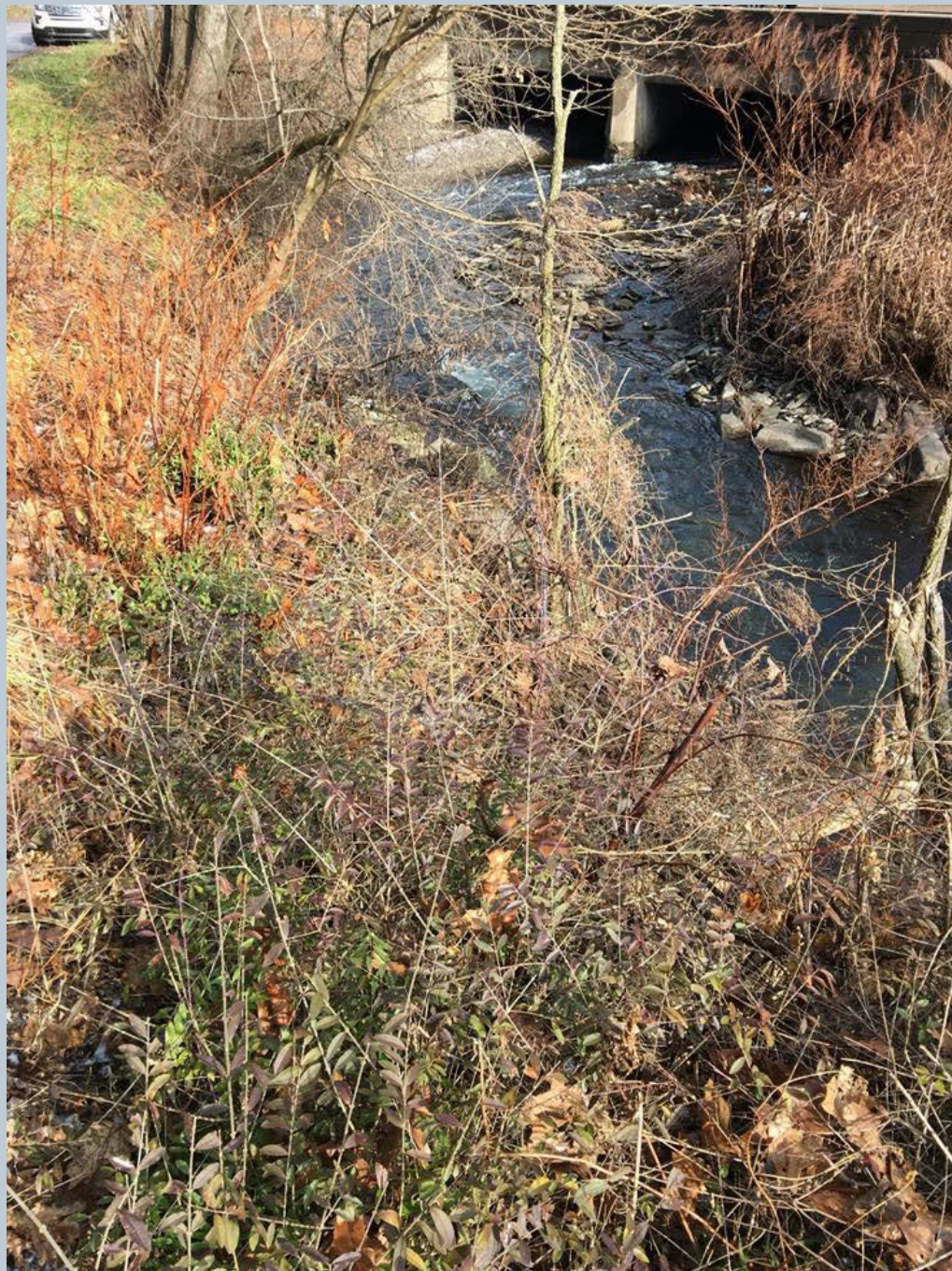
Figure 100. A shot looking upstream at a vertical bank, which has been estimated to be about 12 feet high, along the left bank along S. Main Street. This location is ideal for fishing; this could be a future location for sampling and electroshock surveying.
