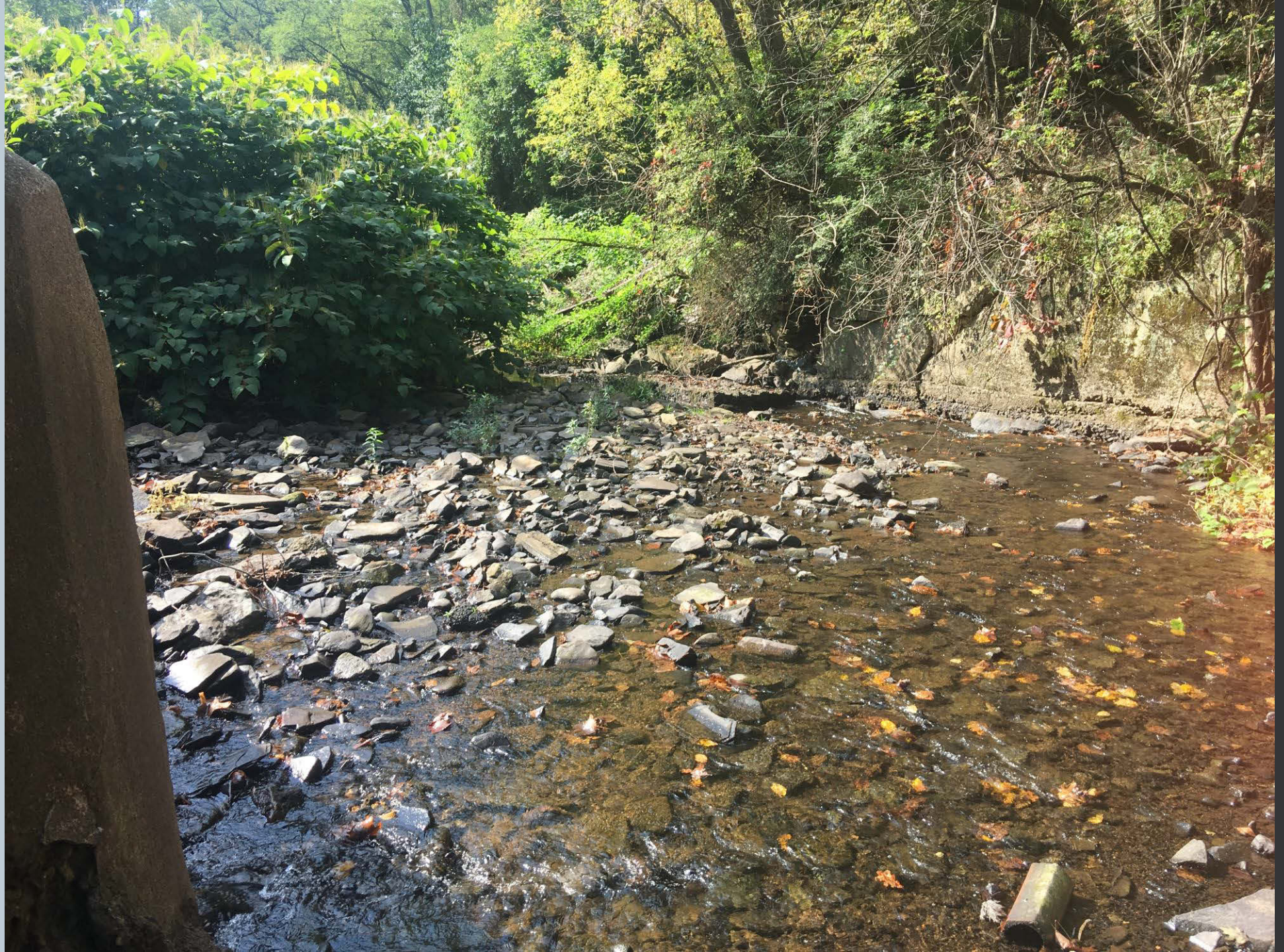
Figure 360. Looking downstream on Toby Creek near Modern Floors Professional Building from the outlet of one of the structures from the bridge culvert over the Dallas Memorial Highway.
